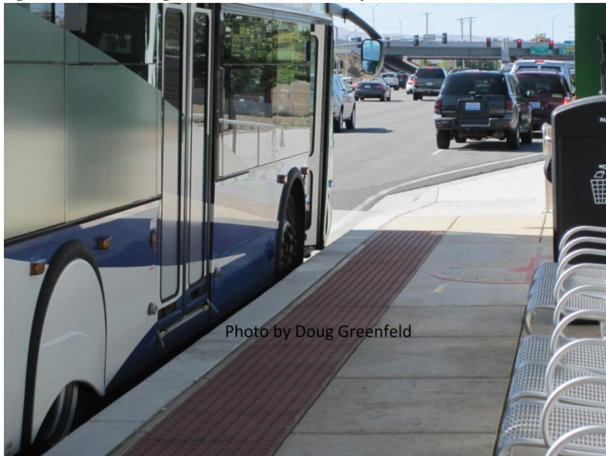
Figure 4: Level Boarding and Bus Bulb on the BRT System in Reno, NV
