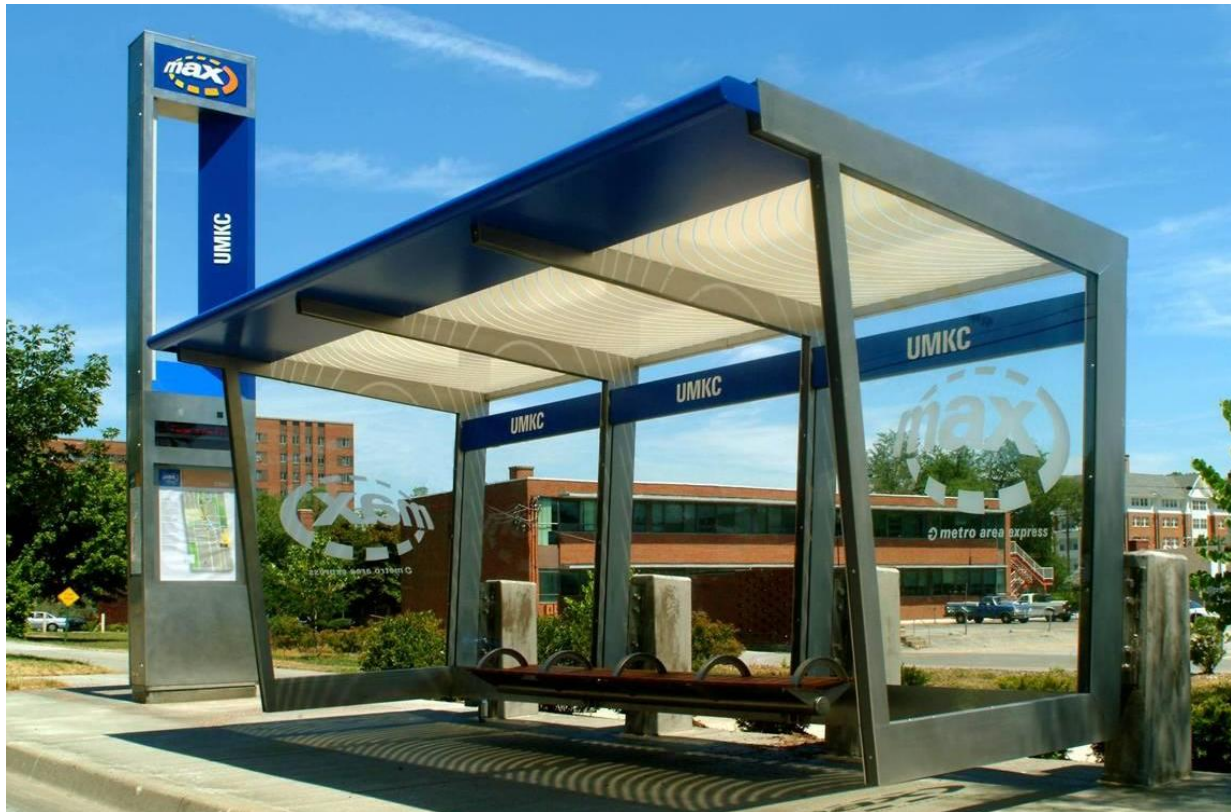
Figure 3: Example of an Enhanced BRT Stop in the Kansas City (MO) MAX System
