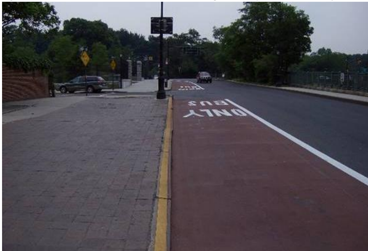
Figure 1: Curb Bus Lane Located within a Street Right-of-Way in New York City
